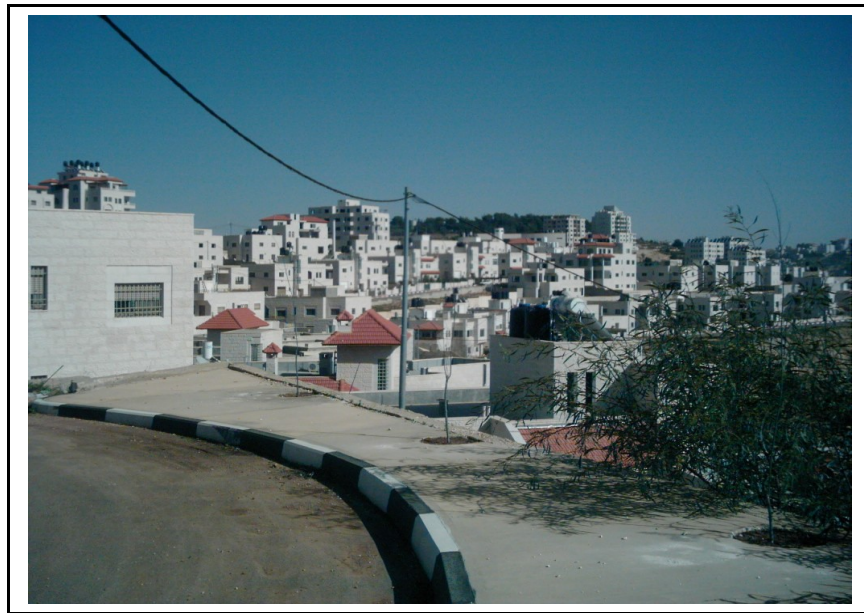
Figure 4 Overview of Attira housing project
